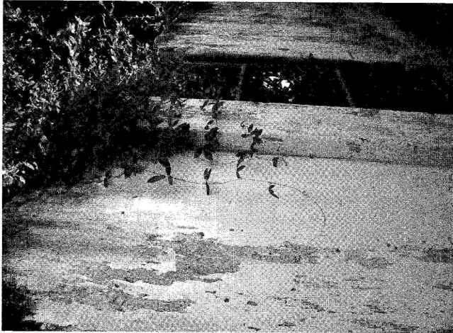
Figure 3.3. Private gate for one of the gardens on Dawn Street.
